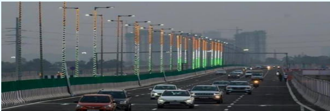
Urban Extension Road (UER II), part of Dwarka Expressway (Pic Via X)
