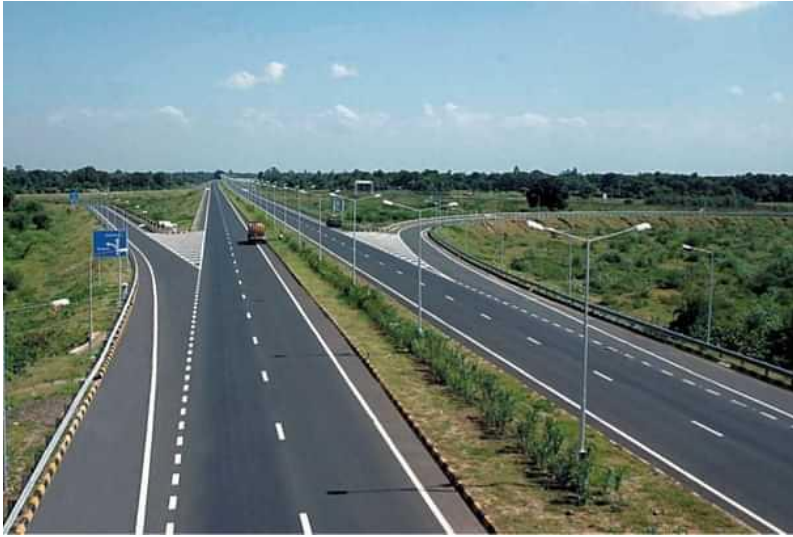
Lucknow is under implementation of various infrastructure projects.
