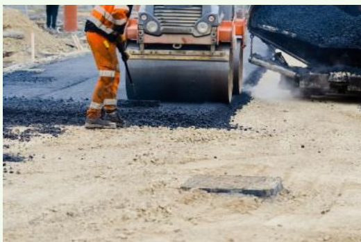
Construction workers in high-visibility gear are applying fresh hot asphalt to roadway surface
