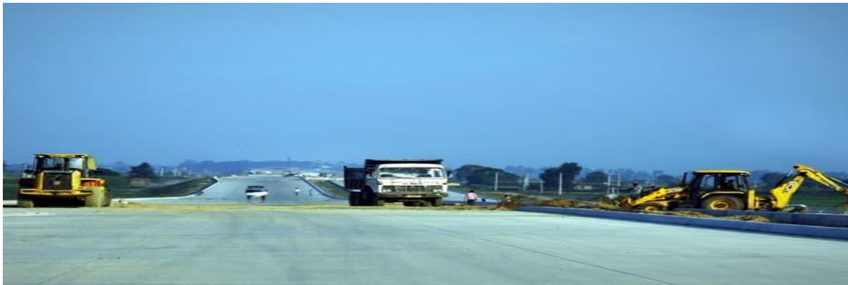
Highway construction in full throttle. (Sonu Mehta/Hindustan Times via Getty Images)
